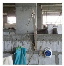
Figure: Workers had tapped into electricity on the construction site to install bulbs near their living spaces in the under-construction building
