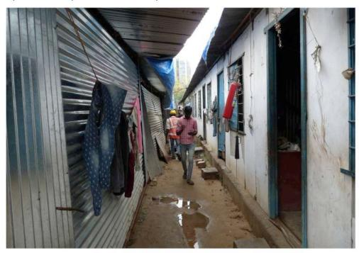
Figure: The construction company had built two types of rooms – one from corrugated metal sheets (left), and the other using Aerocon sheets for the external walls (right).
