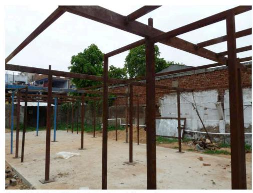
Figure: Fabrication of the structure using metal box sections
