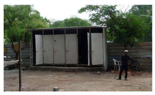
Figure: Men's toilet block built from corrugated metal sheets
