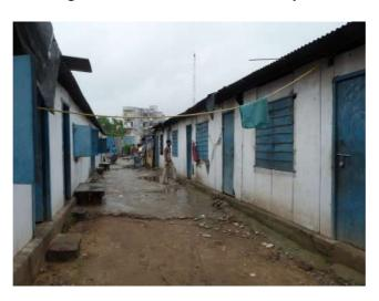
Image 5. Rooms made from Aerocon panels
