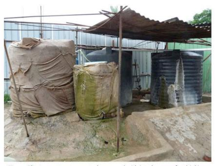
Figure: The two water storage tanks covered with jute bags are for drinking water. The jute bags are for keeping the water cool in the summer.
