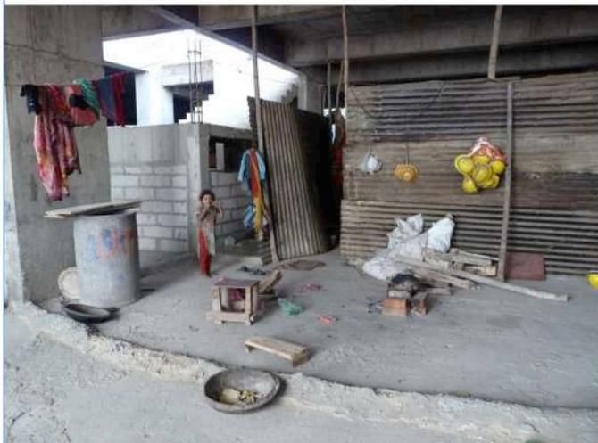
Figure (above): Room-like enclosure made by workers using bamboo and corrugated metal sheets
