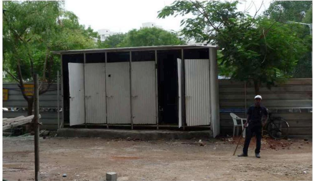
Figure: Men's toilet block built from corrugated metal sheets
