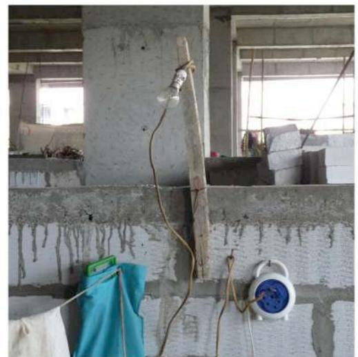
Figure: Workers had tapped into electricity on the construction site to install bulbs near their living spaces in the under-construction building
