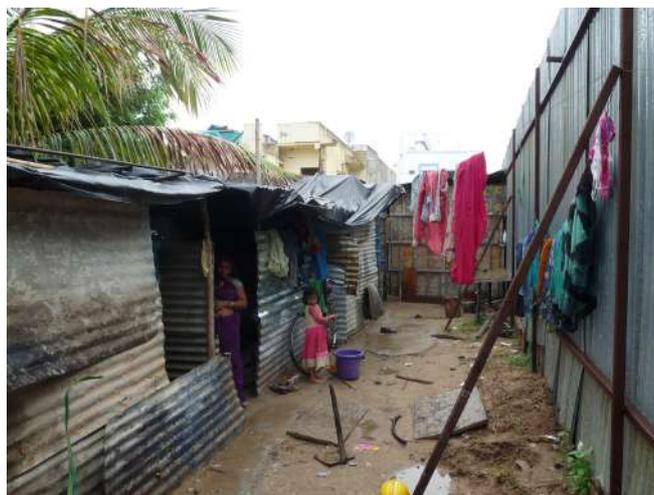
**Image 2 (left). Frame structure made by fabrication onto which corrugated metal sheets are bolted**
