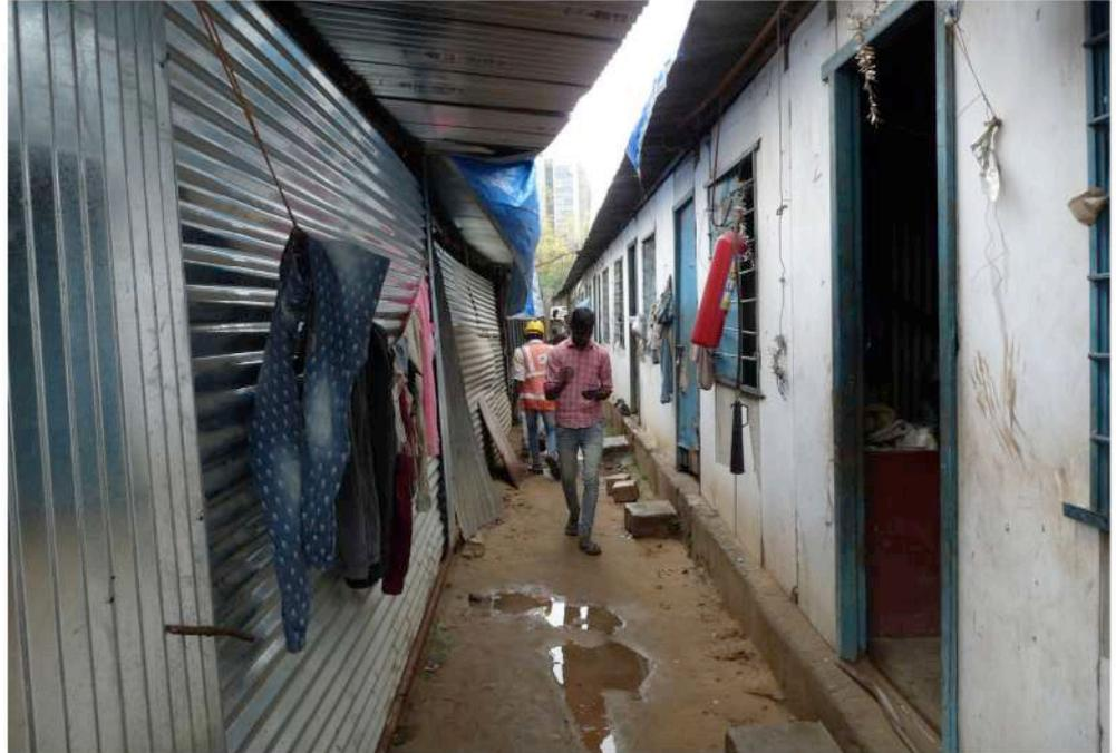
Figure: The construction company had built two types of rooms – one from corrugated metal sheets (left), and the other using Aerocon sheets for the external walls (right).
