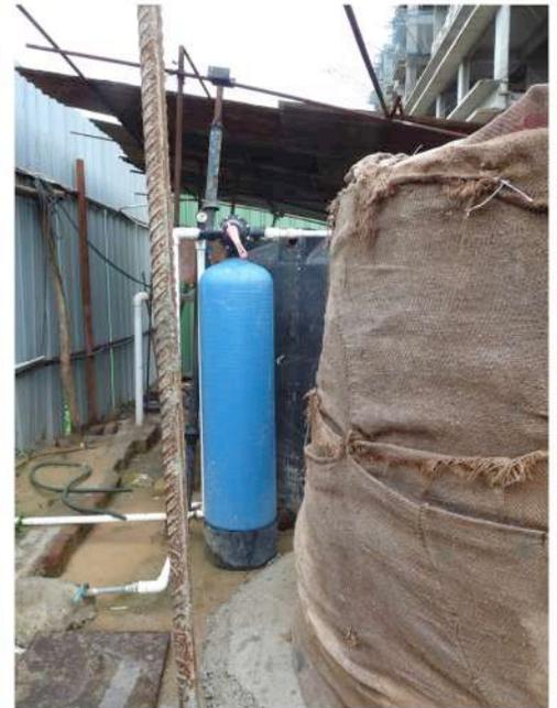
Figure: Filtration system installed for drinking water
