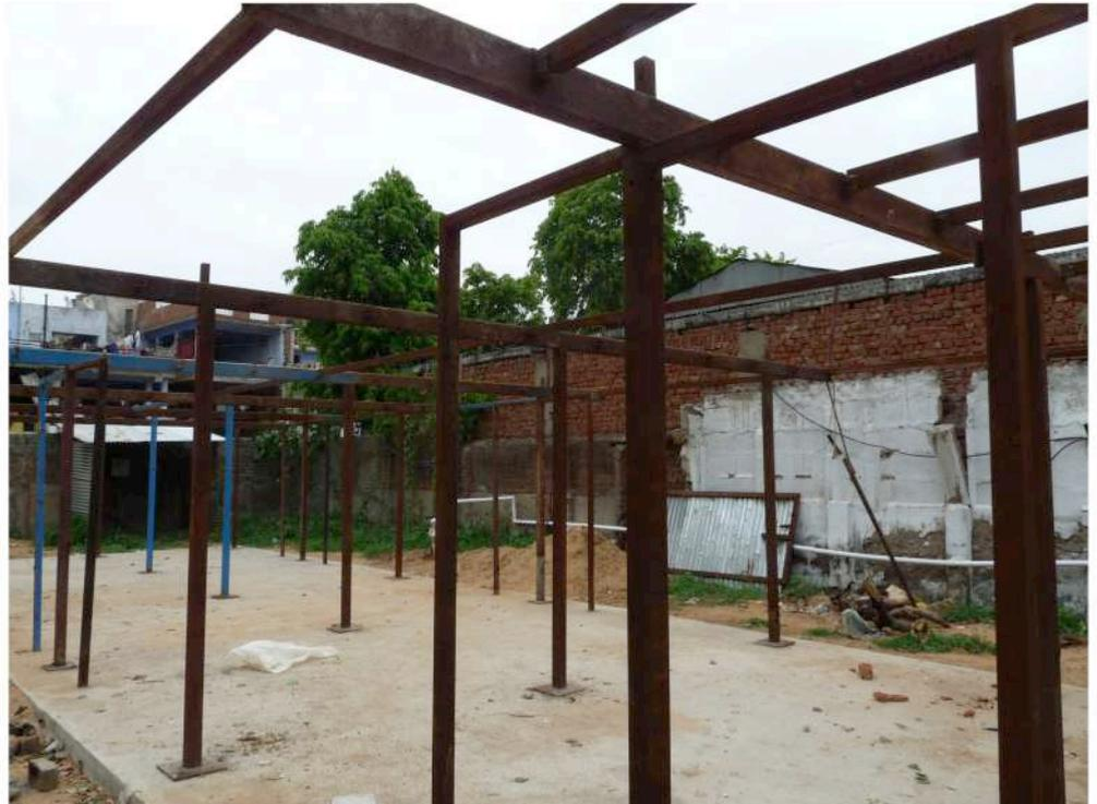
Figure: Fabrication of the structure using metal box sections
