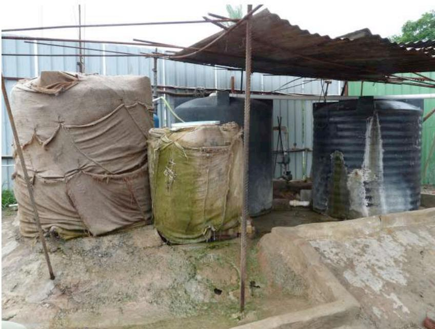
Figure: The two water storage tanks covered with jute bags are for drinking water. The jute bags are for keeping the water cool in the summer.
